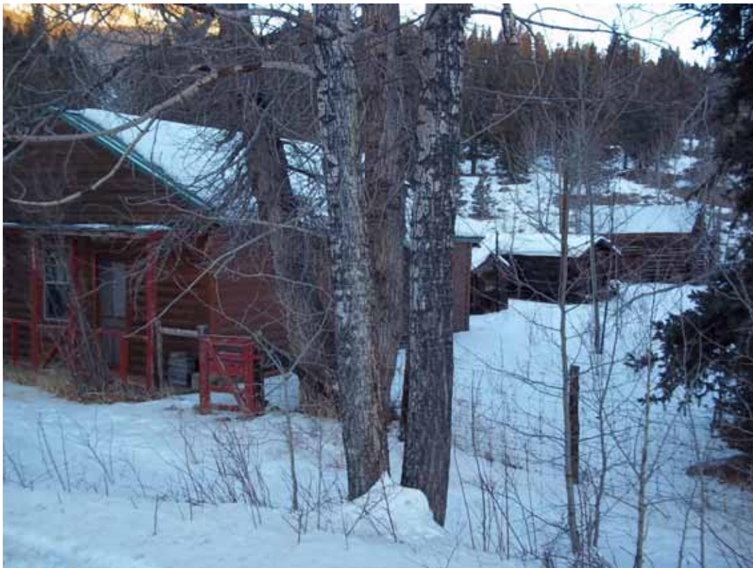
5LK2463, Complex, View to NW, Photo TL-9-3:12
