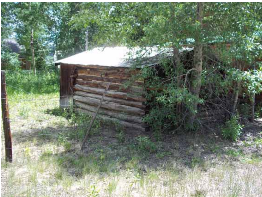
5LK2463, Feature 2 (Ice House), View to SE, Photo TL-9-3:4
