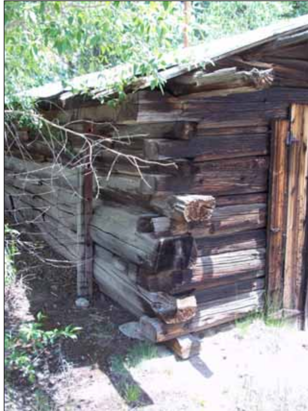
5LK2463, Feature 4 (Garage, Corner Joining), View to SE, Photo TL-9-3:8
