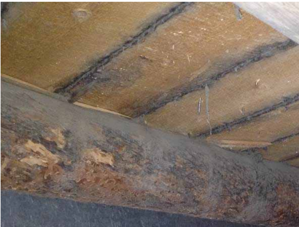
Photo 3.3-2: Top of log is shimmed where floor decking bears
