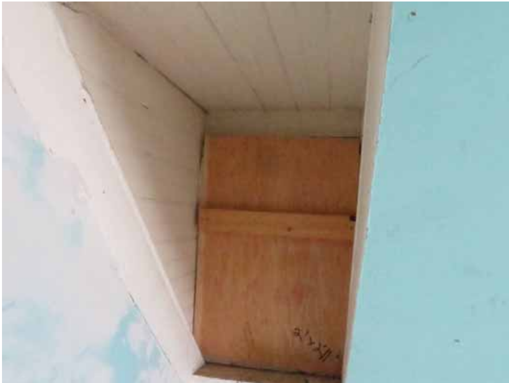
Photo 3.6-4: Dormer in South Bedroom
