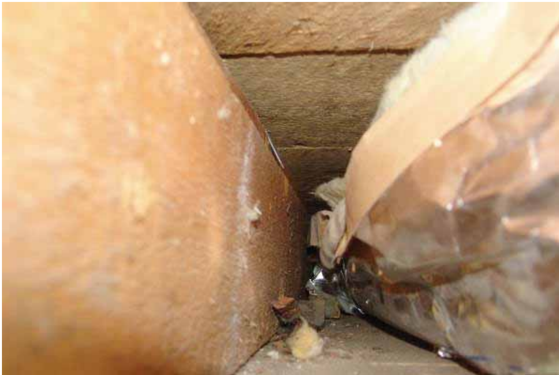
Photo 3.3-5: Second floor joists
