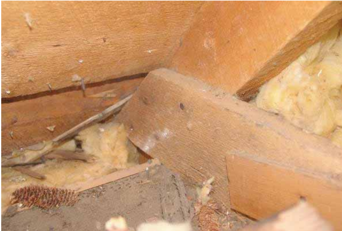
Photo 3.3-15: Main building rafter to collar tie connection with four side nails.
