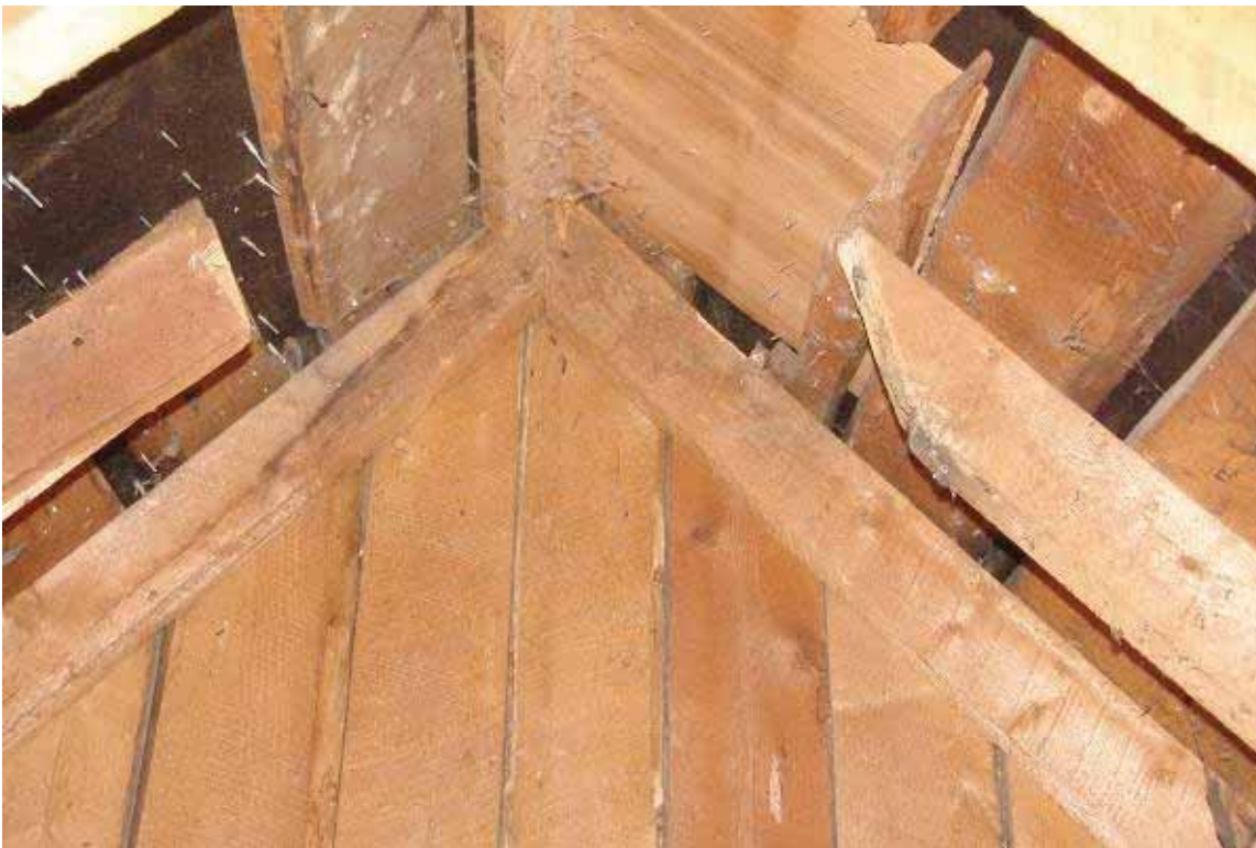
Photo 22: Cut rafters at former roof penetration locations
