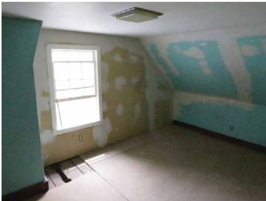
Photo 3.7-5. South bedroom looking southwest
