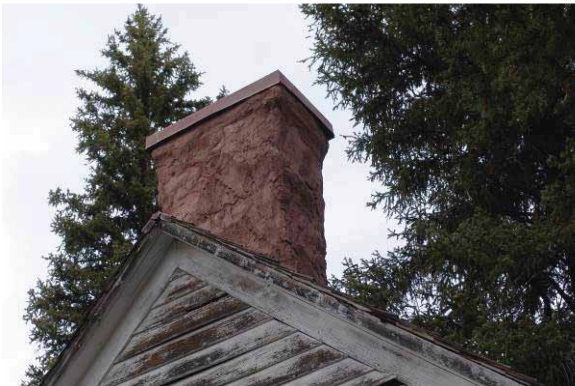
Photo 3.4-9: Adobe chimney above roof
