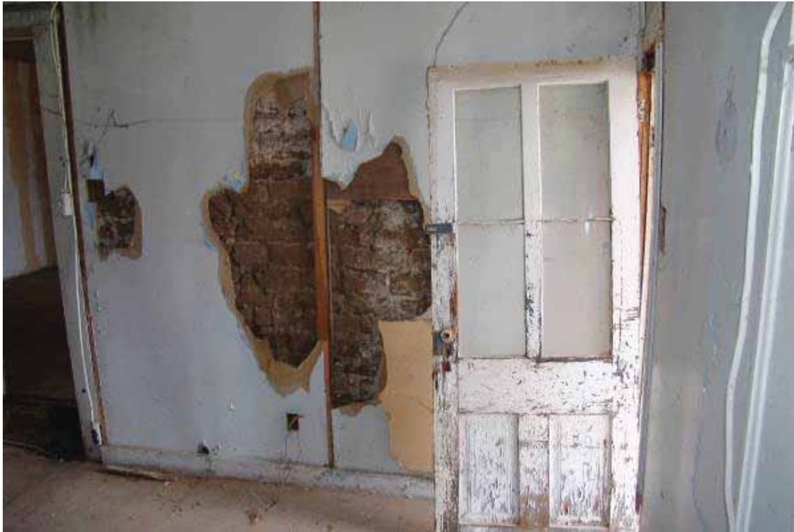
Photo 3.4-6: Adobe wall on south elevation of main building. Looking north inside Room 3
