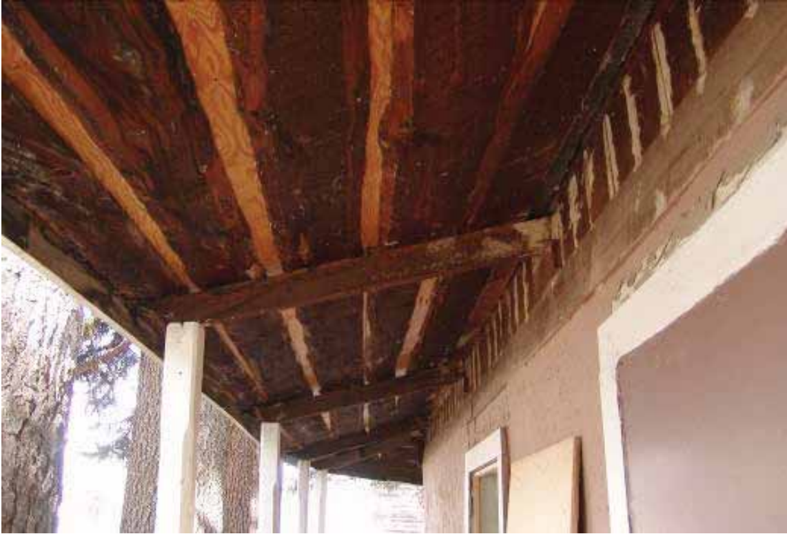
Photo 21: Underside of the porch roof framing
