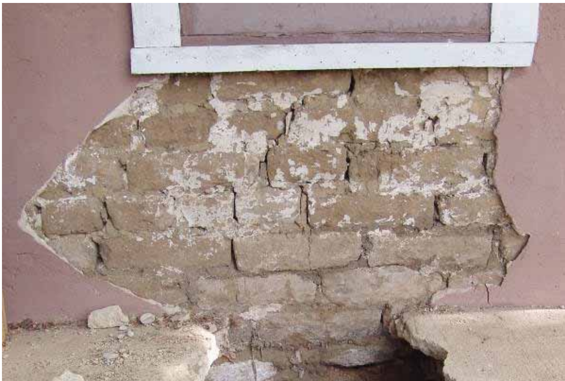
Photo 3.4-5. Adobe wall on north elevation
