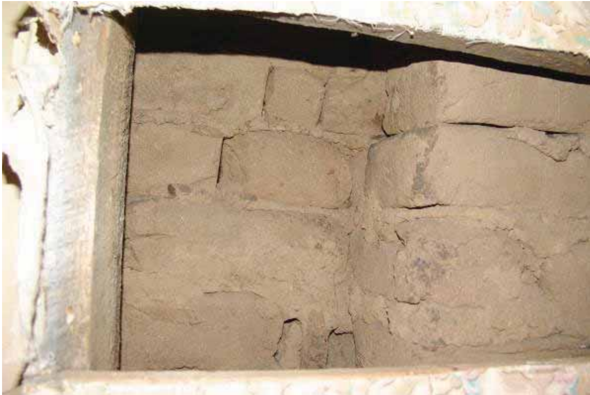
Photo 3.4-8: Adobe chimney behind furring wall on first floor inside Room 2
