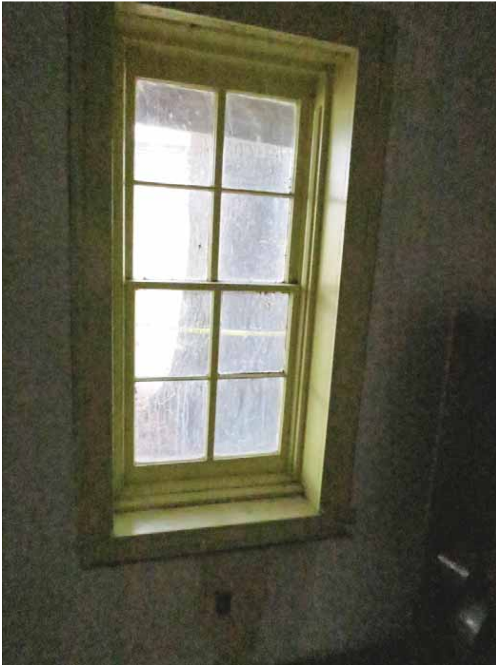
Photo 3.6-2. First floor, east side, interior
