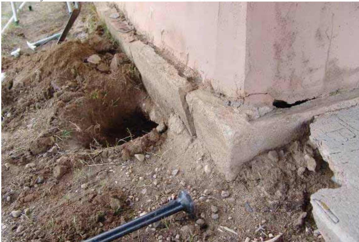
Photo 3.2-8: Concrete curb/parge coat along base of south addition exterior walls
