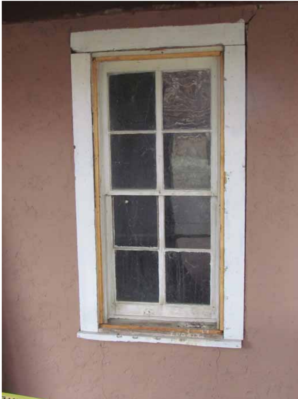
Photo 3.6-1. First floor, east elevation, exterior of window
