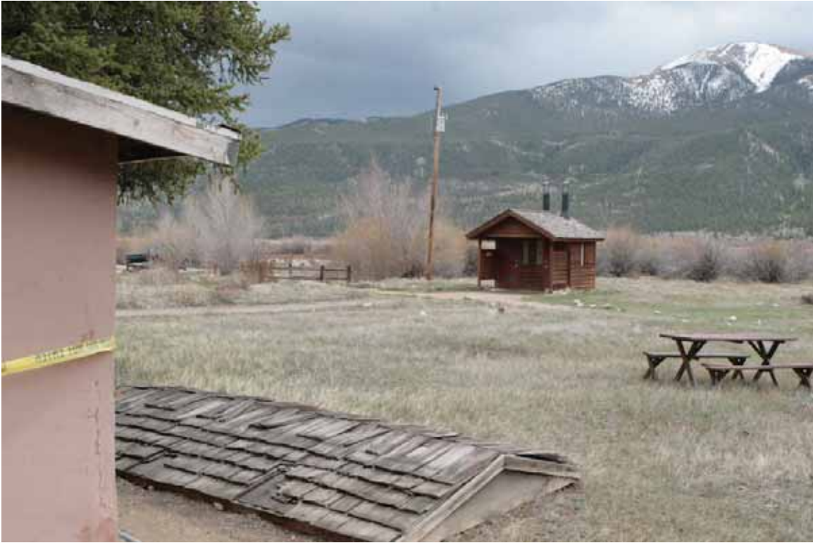
Photo 3.1-2. Looking southeast at wetlands and non-historic toilet building. Just south of the Clarion, a shallow gabled roof with wood shingles covers an unused storage pit.
