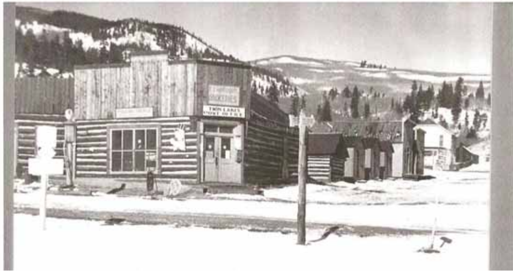
Photo 2-3. This photograph shows the north face of the general store owned and run by E.J. Hofenagel. The General Store was one block east of the Clarion Hotel. The proprietor's sign is above the Twin Lakes Post Office sign on the corner of the building. A Shell gasoline sign is to the right of the front door and a gasoline pump is to the left of the store windows. The Post Office operated in the General Store until 2011. Photograph courtesy of Twin Lakes Visitor Center.
