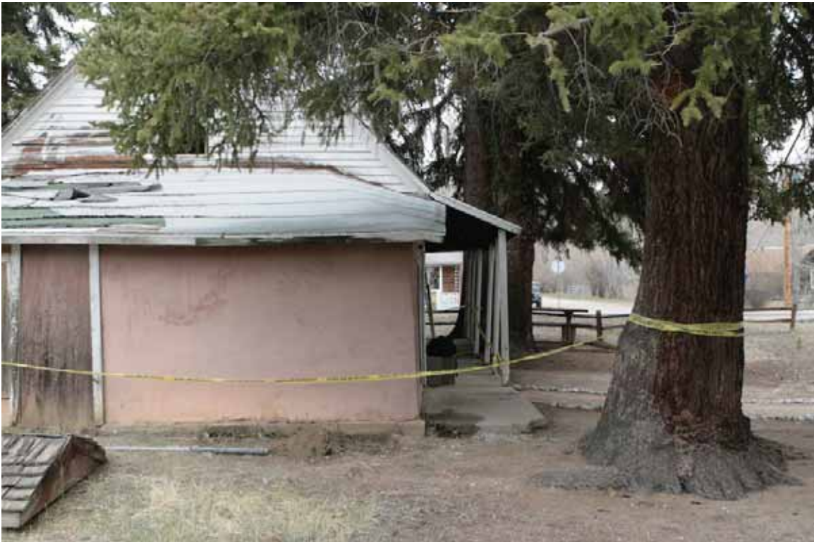
Photo 3.1-3. Site along south and east sides
