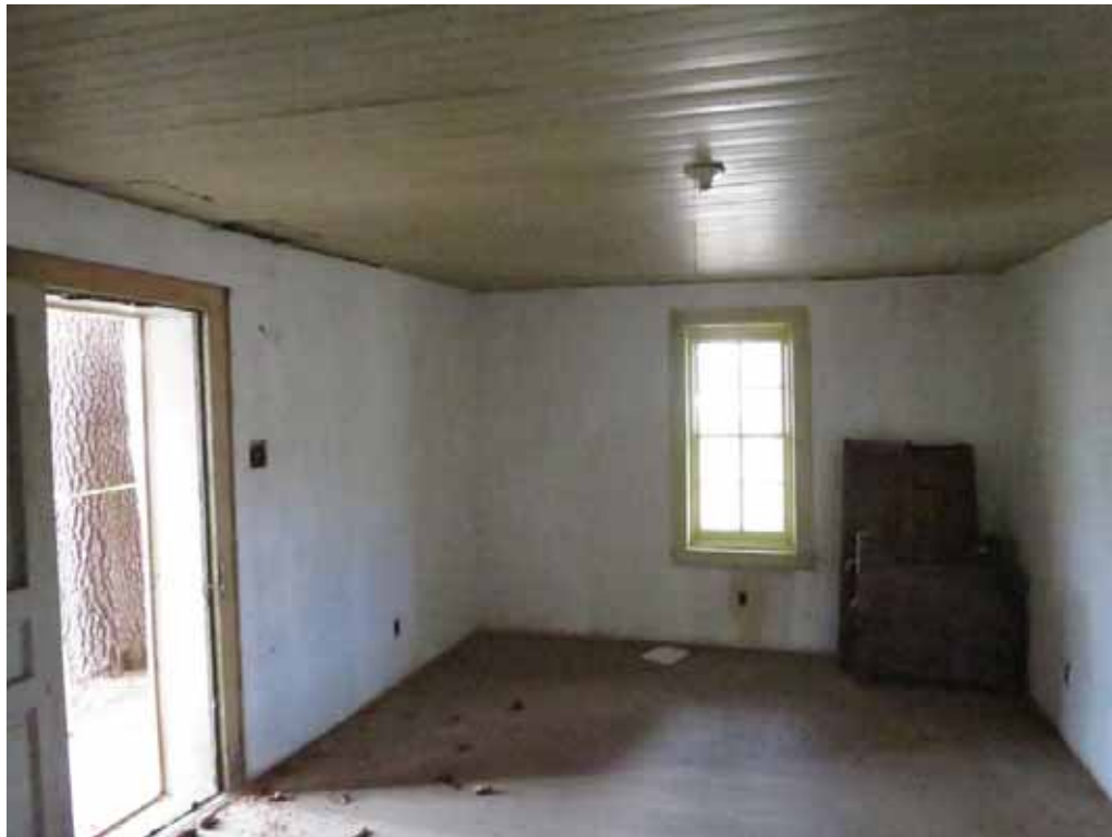
Photo 3.7-1. Room 1, looking east.
