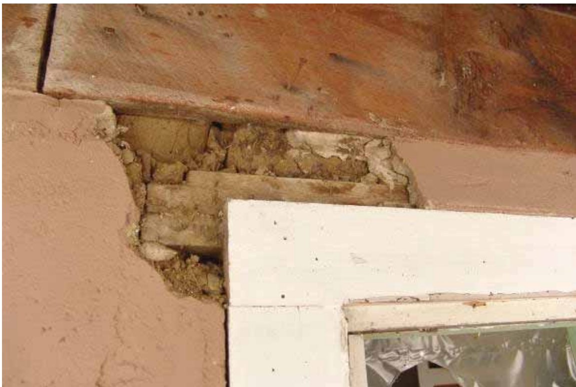
Photo 3.4-7: Flat wood lintel embedded in adobe assembly along east elevation
