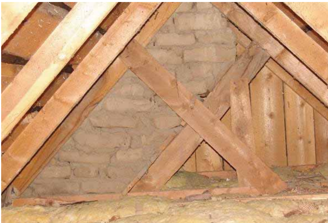
Photo 3.3-16: Struts supporting battered adobe chimney at south end of attic
