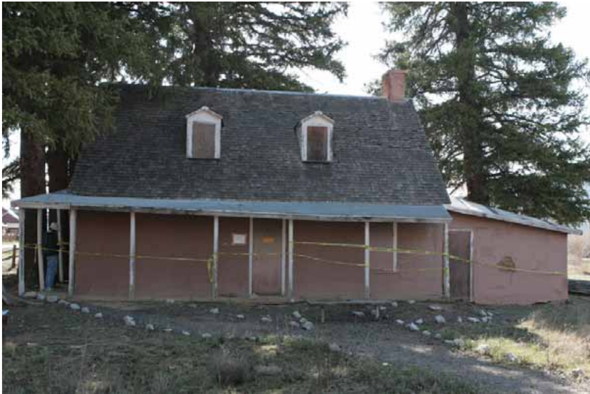
Photo 2-9. 2014 photo of west side
