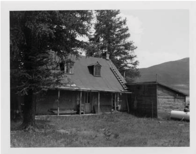
Photo 2-15. 1974 National Register nomination photo shows two dormers and a shed-roofed structure with wood siding on the south side of the main building. The nomination notes that the building has brick facing.
