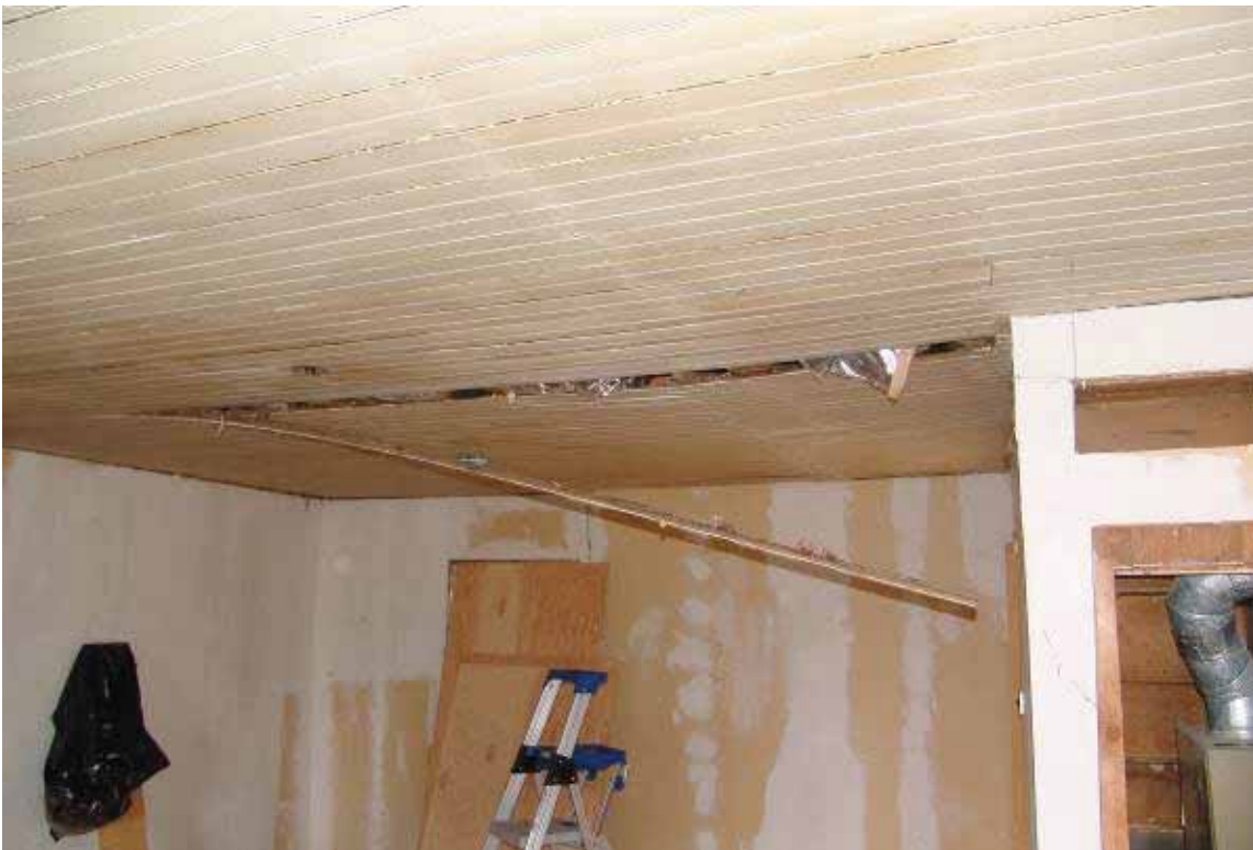
Photo 3.3-8: Bead-board ceiling finish on the underside of the second floor joists, Room 2
