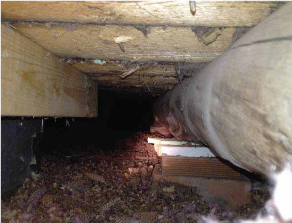
Photo 3.2-5: Isolated adobe, wood, and miscellaneous material log joist support in the north framing bay
