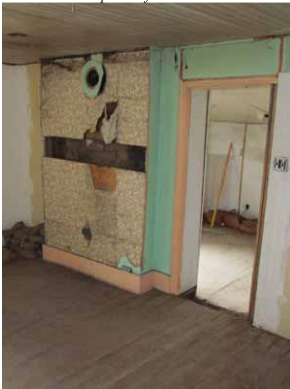
Photo 2-10, looking southeast in room 2: beadboard ceiling, board flooring, adobe chimney
