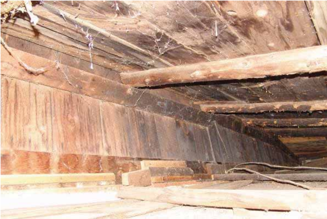
Photo 3.3-17: Ceiling joists and rafter ledgers at south lean-to addition above Room 3
