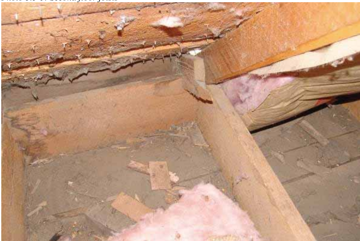
Photo 3.3-6: Second floor joists bearing on adjacent plates over adobe wall. Note also rim board, rafter, and back of porch rafter notched over rim board
