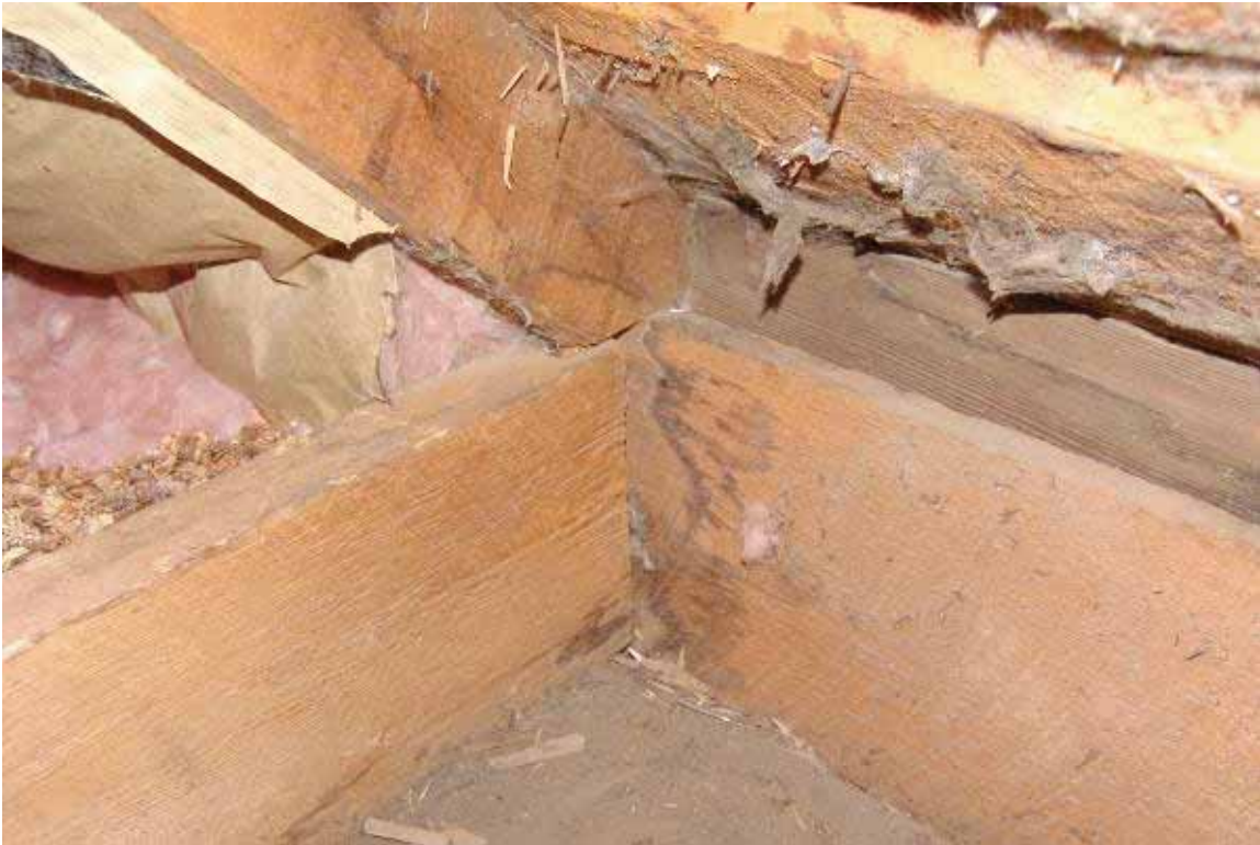
Photo 3.3-13: Main building rafter to joist connection with four side nails.
