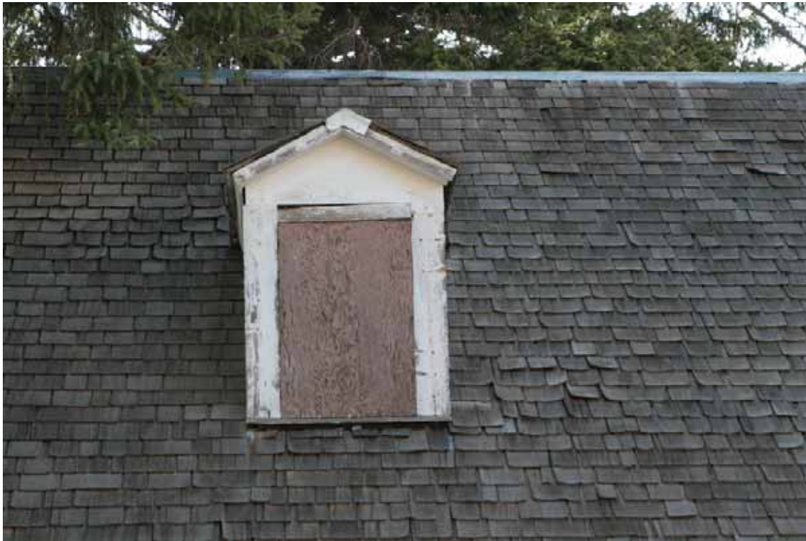
Photo 3.6-5: East side dormer
