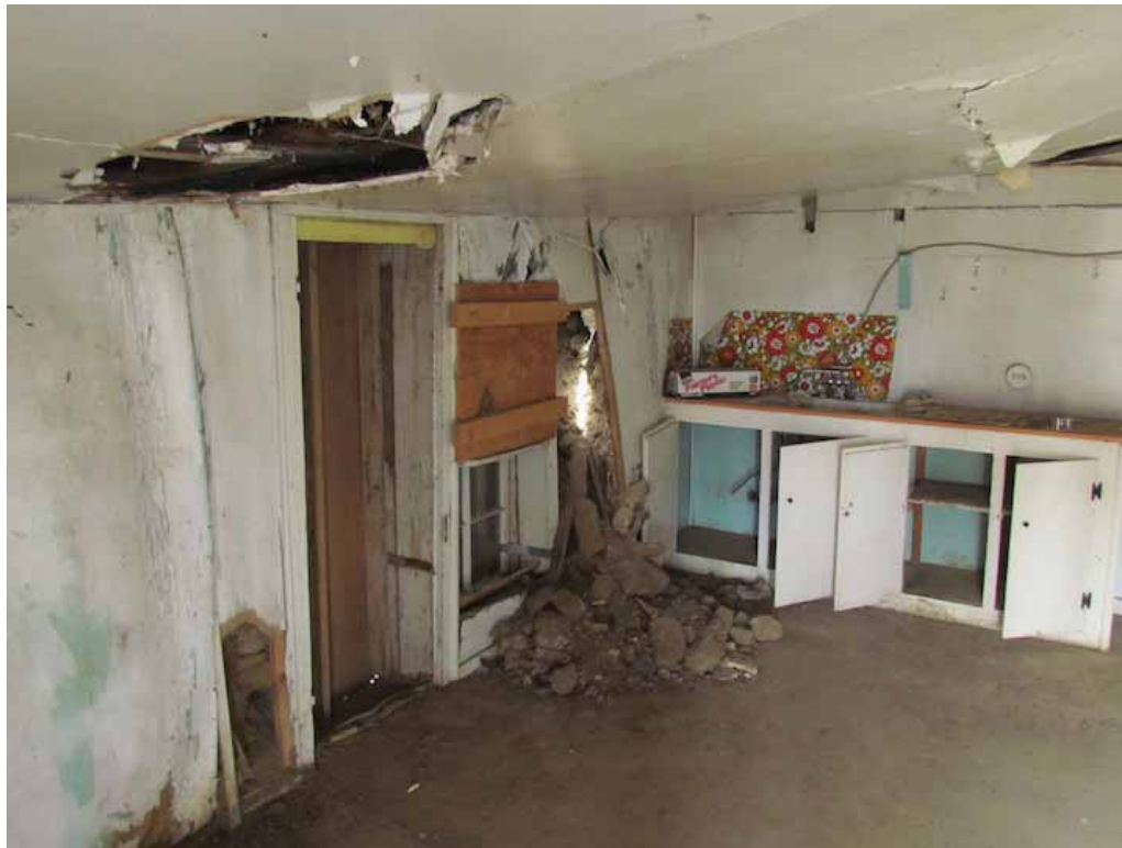
Photo 3.7-4. Room 3 looking southwest.
