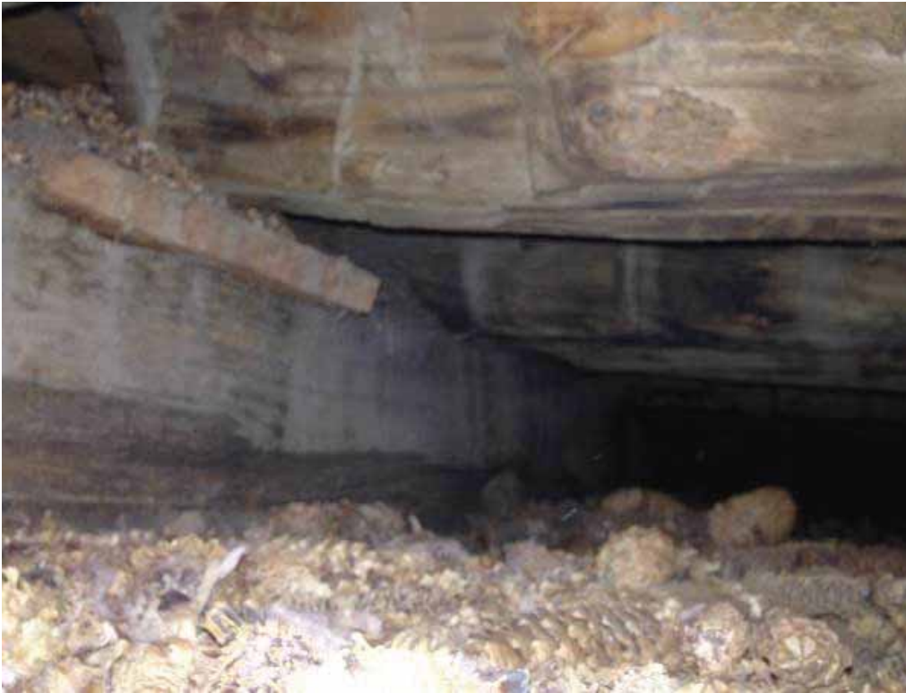
Photo 3.2-3: Log sill/foundation dividing north and south first floor framing bays
