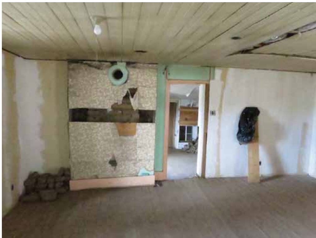
Photo 3.7-2. Room 2, looking south.
